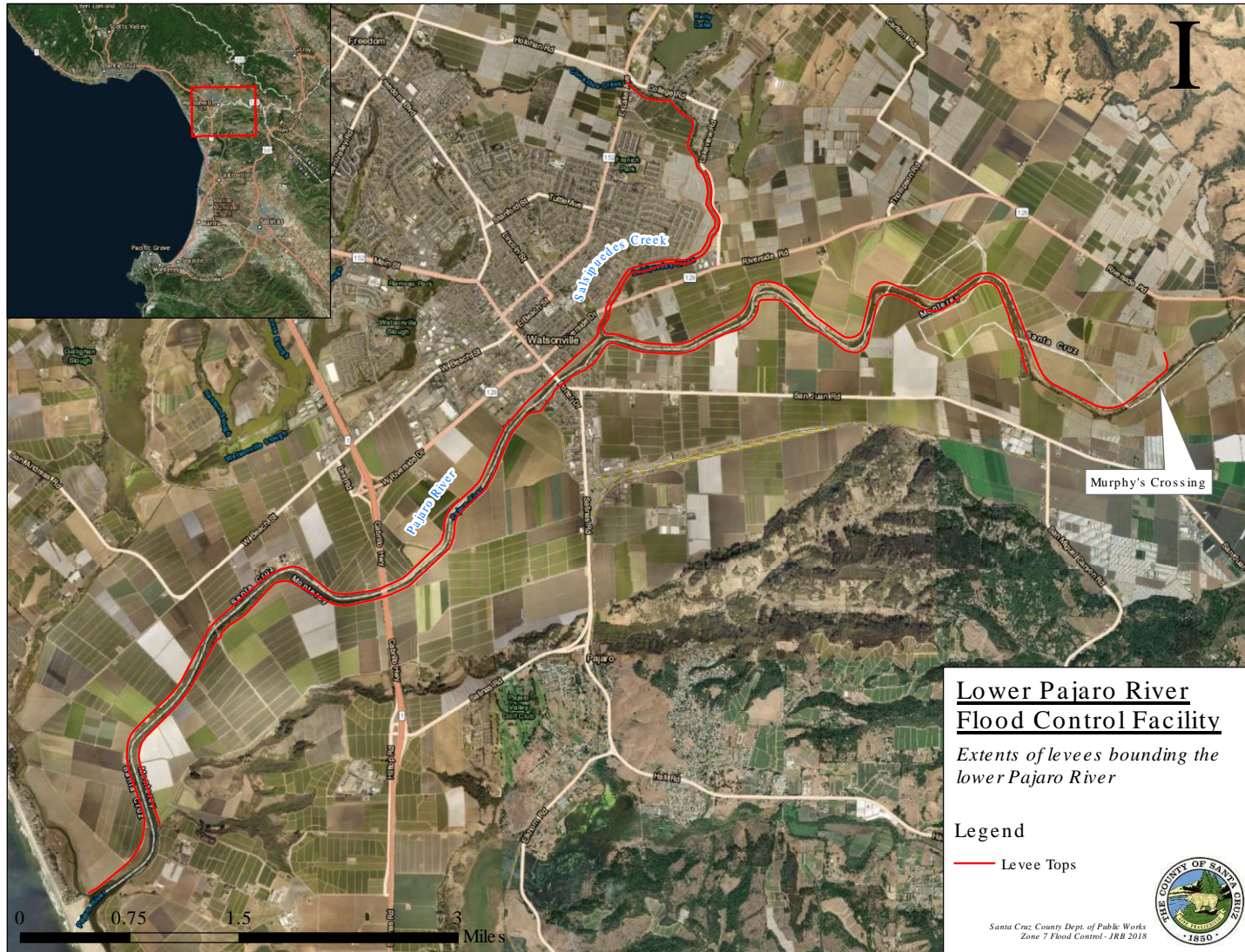
Figure 6—Lower Pajaro River Levee Patrol Area (Zone 7 only responsible for levee reaches within Santa Cruz County)
